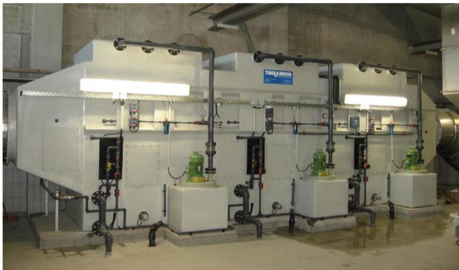
Figure 2 3-Stage Cross-flow scrubber
